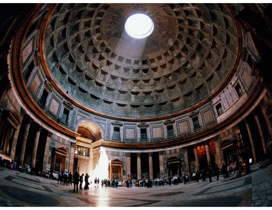
The dome weighs five thousand tons. It is the largest unreinforced concrete dome in the world, and in history. We can't built a bigger one today.
